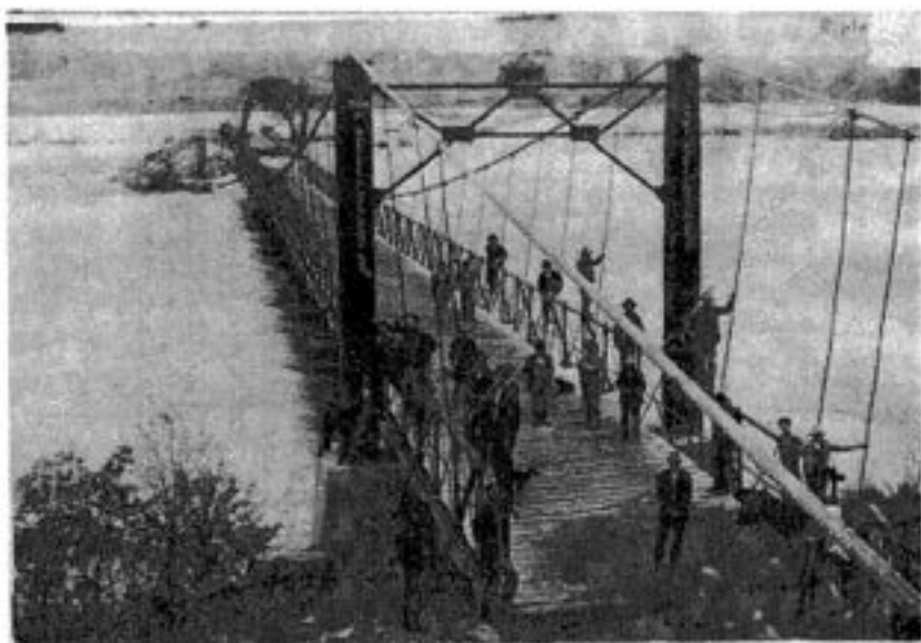
Ripley's suspension bridge over the Cimarron River, built in 1909, was damaged in the flood of 1912.
