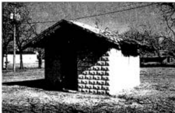
One of Stillwater's historic landmarks is this well house built by Charles Donart on his farm homesteaded in 1889. It is just south of the Southside Baptist Church on Perkins Road. Photo courtesy of D. Earl Newsom.
